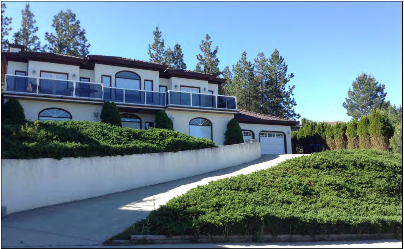
Figure 14. Hazardous landscaping of an interface home. Note sprawling juniper hedge, 3 m tall cedar hedge to the right and directly against the front of the home and under eaves.
